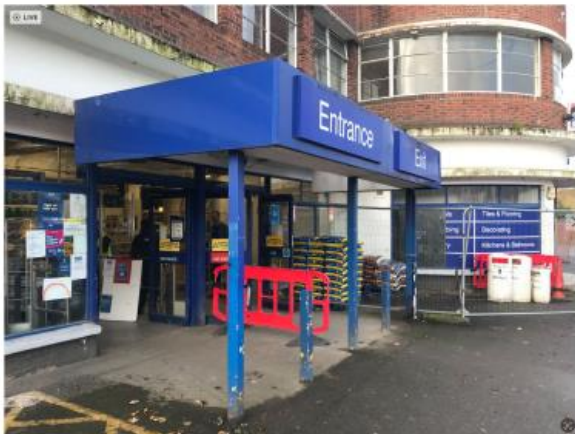
Image 6: Entrance Canopy As Existing
